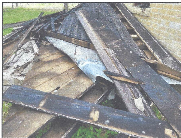
South side of building where metal and wooden debris from roof has fallen. Not suspect ACM.
