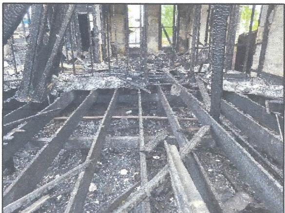
View inside the building showing where the subflooring has burned and fallen into crawlspace. Piping in crawlspace has no insulation. Not suspect ACM.
