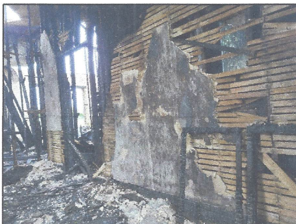
View of rock lath remnants on wall. Photo taken through window on east side of building. The cellar is located below this area. Not suspect ACM.
